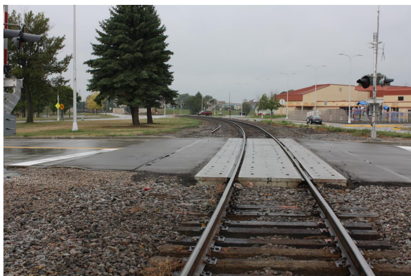
Improved at-grade Railway Crossing- East Grand Forks. Photo © MPO Staff, 2017
