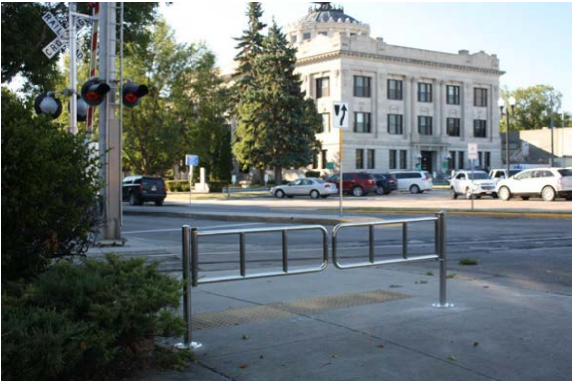
Pedestrian Swinging Gates, Kittson Avenue at S 4 th Street-Grand Forks-- Photo: © MPO Staff, 2017
