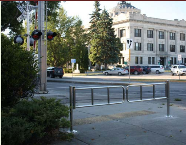
Pedestrian Swing Gates –Kittson at N 4 th Street Photo © MPO Staff, 2017
