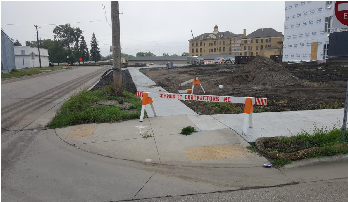
Sidewalk Construction, Photo © MPO Staff, 2017
